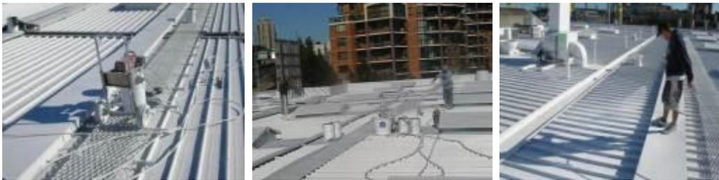
Once the roof was repaired and coating systems applied, it was critical that trades people going onto the roof to undertake maintenance to the plant there or mobile phone towers, did not walk on the roof membrane and damage same. Therefore extensive aluminium walkways were installed throughout the roof.
