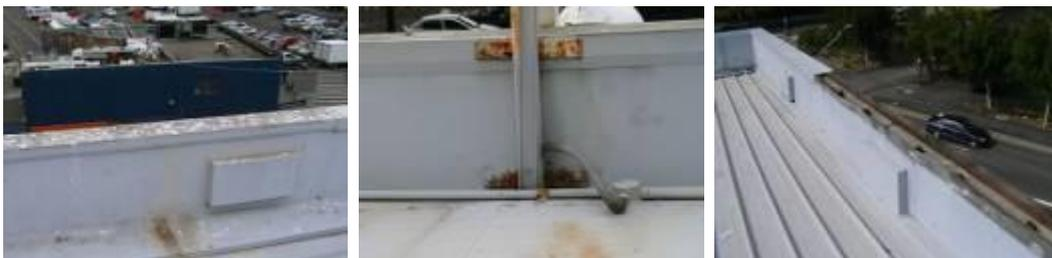
Numerous mobile phone towers were repaired with new flashings and dektites as the existing ones had perished from the continued exposure to water and bird droppings.
