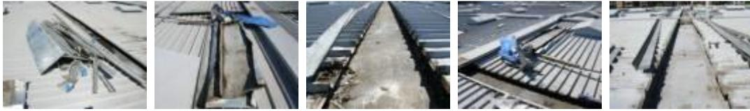
The sheeting profile has not been available for many years so replacement sheeting for those badly corroded areas was not available. In those areas and all holes/rust-affected areas, the rust was treated and the damaged/rusted areas and numerous holes were fibreglass/membrane patched prior to the main coatings being applied.
